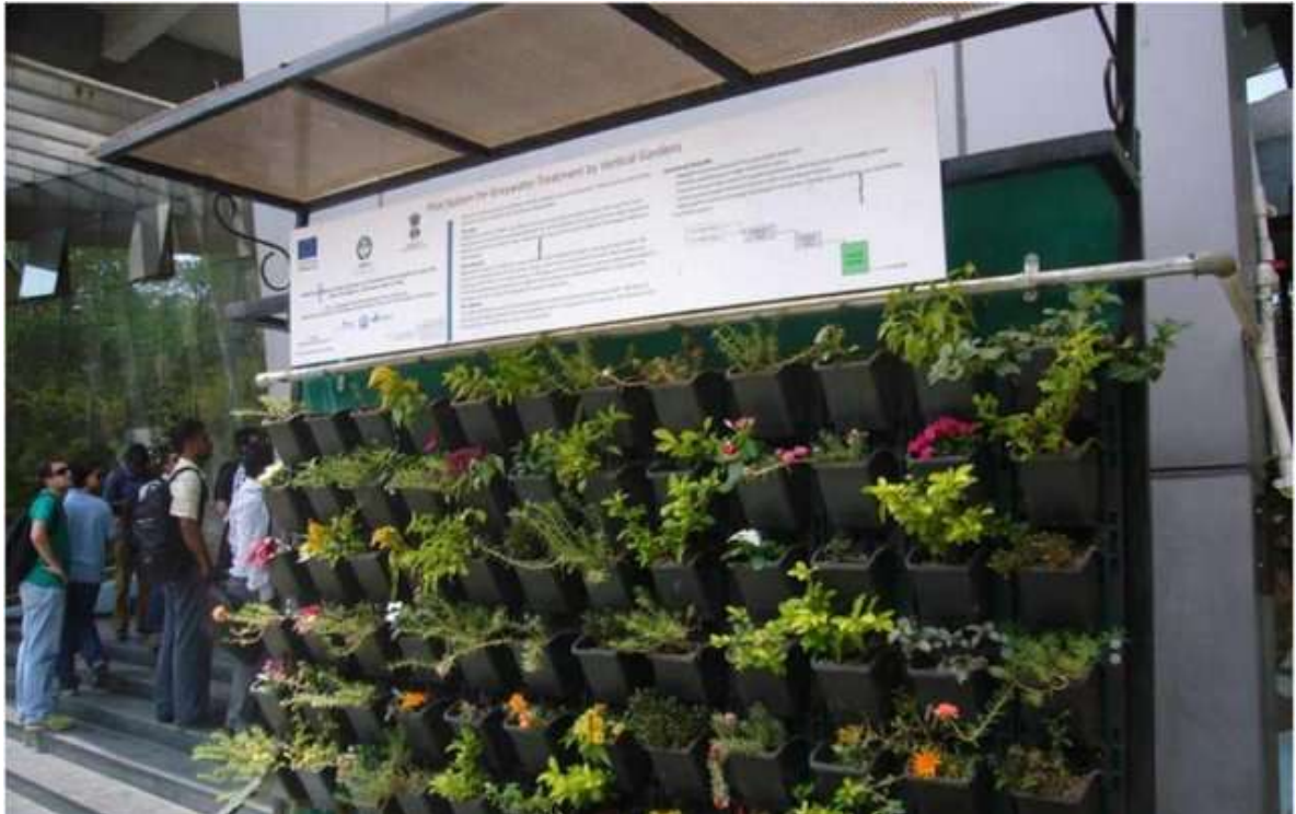
Figure 4.2.6: Living walls installed at the Maharashtra Jeevan Pradhikaran office, Pune (Source: Masi et al., 2016)
