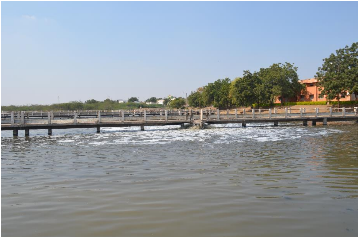
Figure 2-10: 30 MLD capacity Ananthapur Road UWTP
