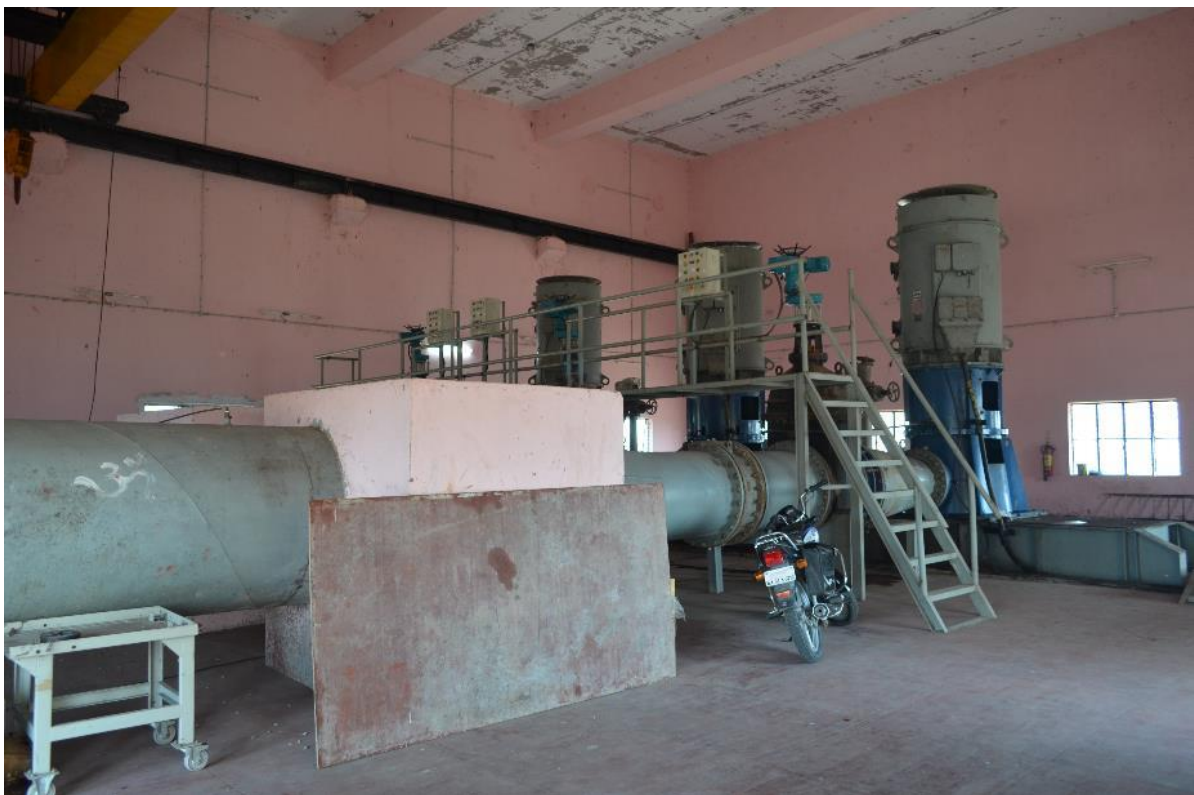
Figure 2-4: LLC Pump house
