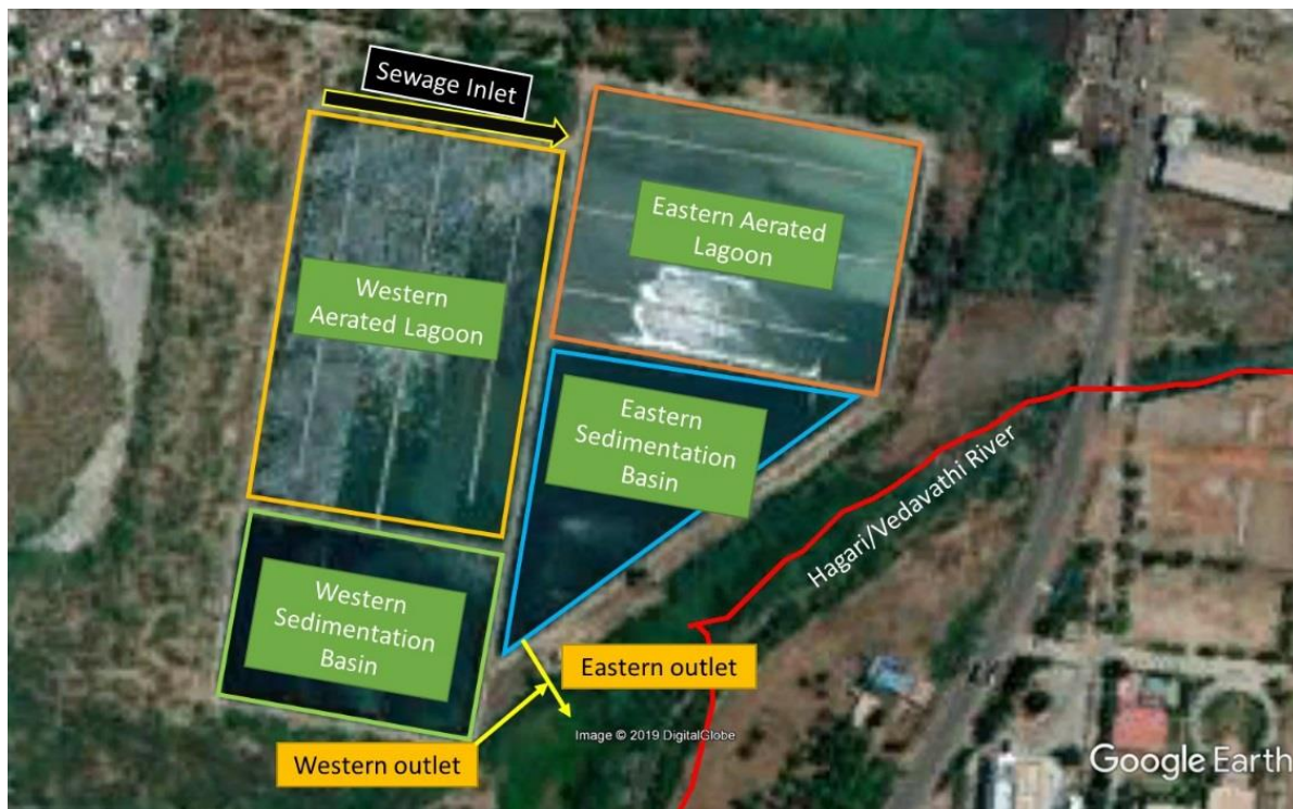
Figure 2-7: Aerial image of 30 MLD capacity Ananthapur Road UWTP
