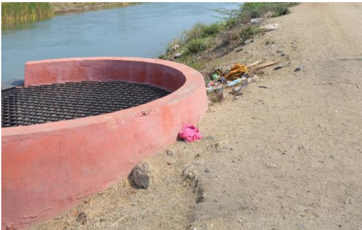
Figure 2-2: Tungabhadra low level canal supplying drinking water to Ballari
