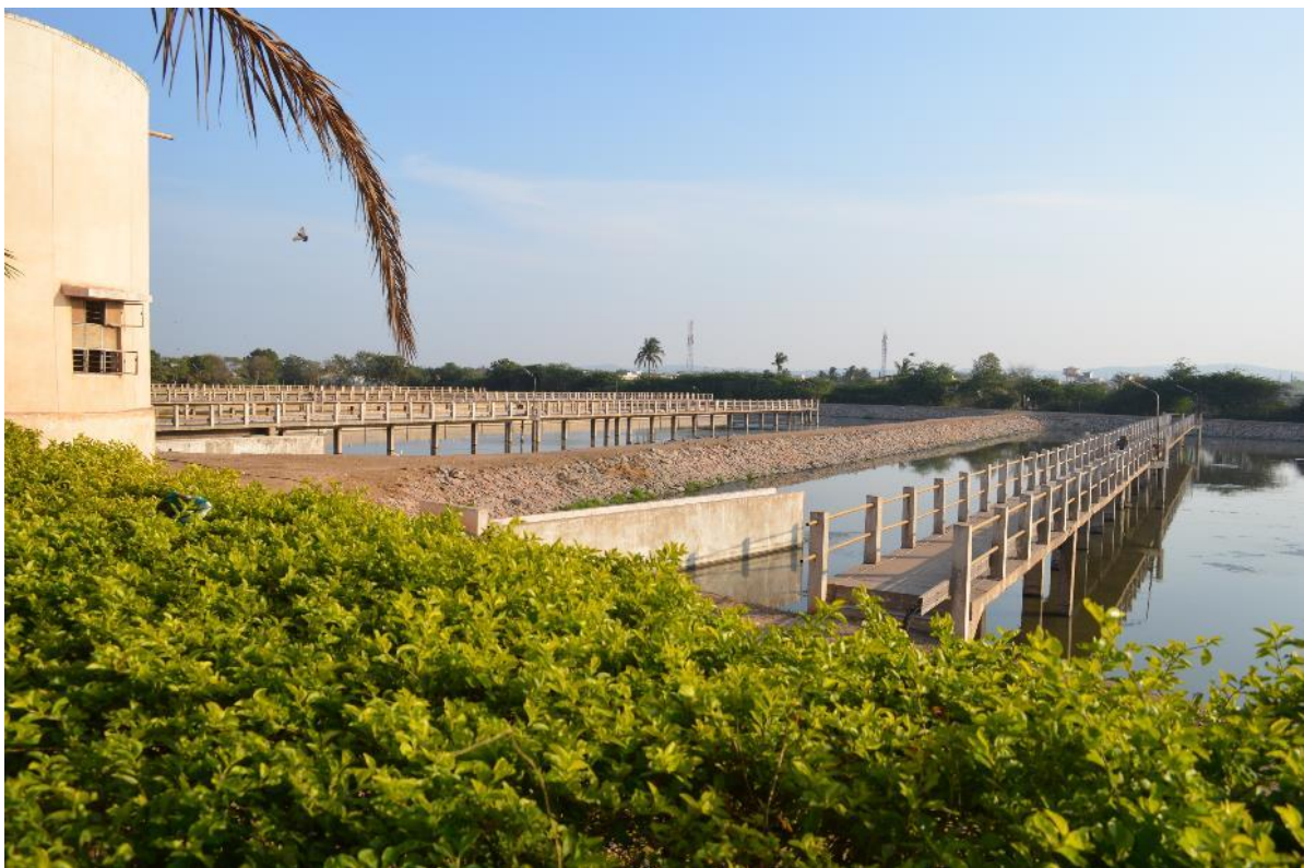
Figure 2-11: 15 MLD capacity Cowl Bazaar UWTP
