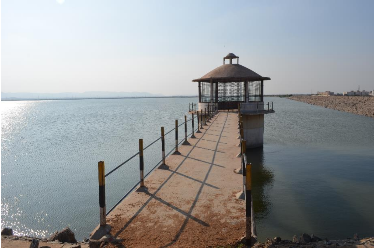
Figure 2-5: Allipura Impounding Water Supply Reservoir
